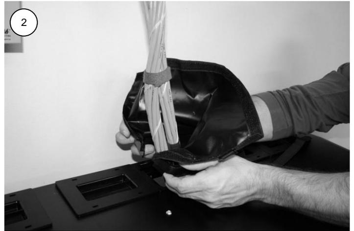
Step 2: Place the fitting around the cable bundle.
